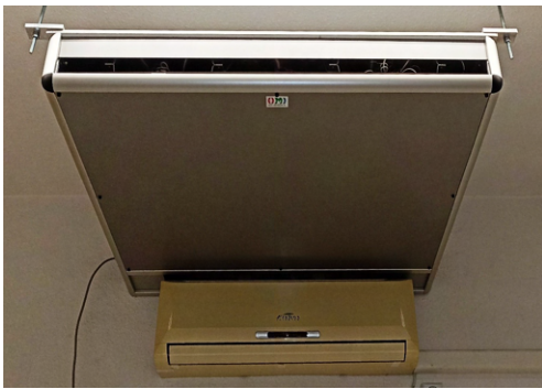
OMI 7-190-000 UV-C air purifier attached to AC indoor unit
